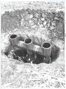
Anlet 306 Anstalled B" to 8" coulfer To stand pips also motalled Gross and two 90° Eltows.
