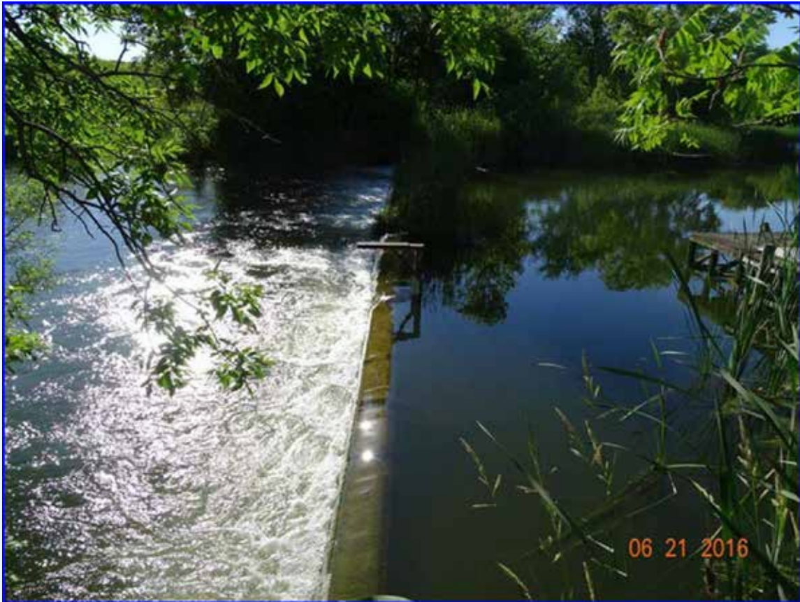
Lake Washington dam in 2016. Note the Carp barrier post and the deflected flow pattern at the post.
