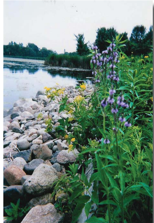
Shoreline stabilized with riprap and enhanced with a vegetative buffer.
